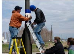
The hardest part was wrapping the sign around the pole and vice-gripping the two ends together.
